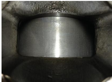
Piston barrel/skirt
